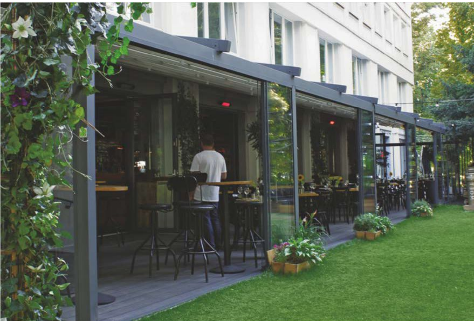
▲ Na Lato Restaurant, Rozbrot 44 A street, Warsaw Production year: 2015, Area: 200 m 2 , Includes: Roof integrated remotely controlled LED light spots (80 pcs.); 5-rail sliding glass system; Infrared heaters (24 pcs.)
